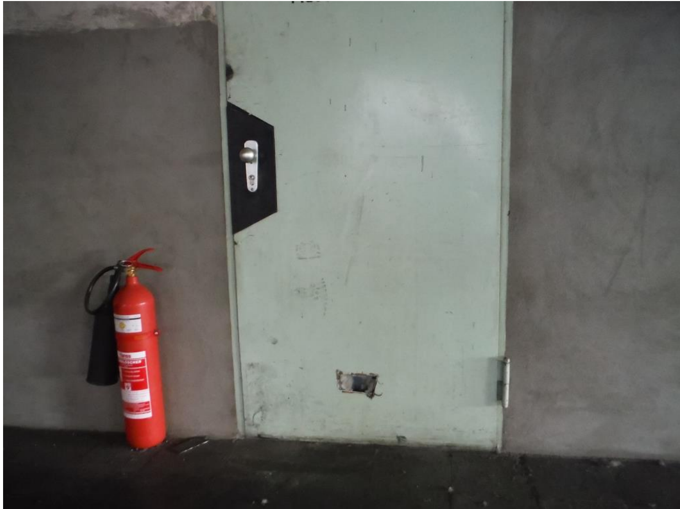
Brandschutztür (Asbest)
